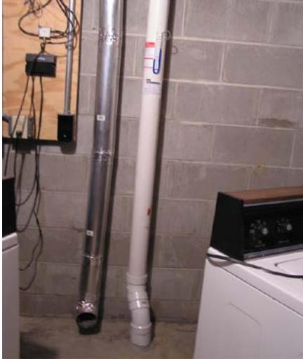
*In this picture, a PVC pipe is connected to an existing drain tile under the foundation of a home. The performance indicator (blue tube) shows the fan is working.*
