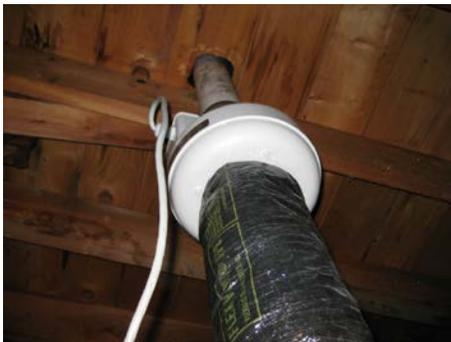
*The radon fan should be located in an unconditioned space, such as the attic or outside. This fan will pull the radon gas from the soil and help expel the gas above the roof line.*
